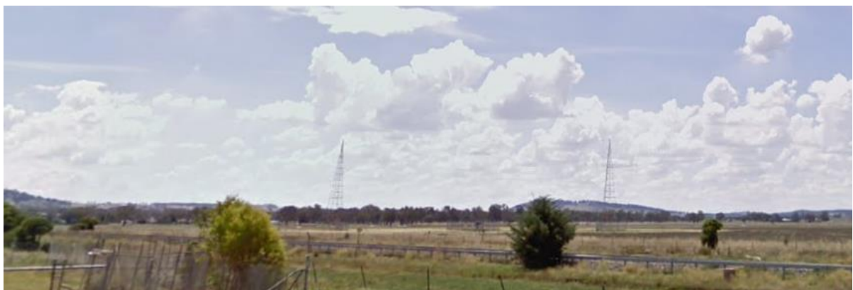
Figure 3 – Redundant infrastructure (towers, hut and contents) to be removed (source: Instantstreetview.com, 2010 )
