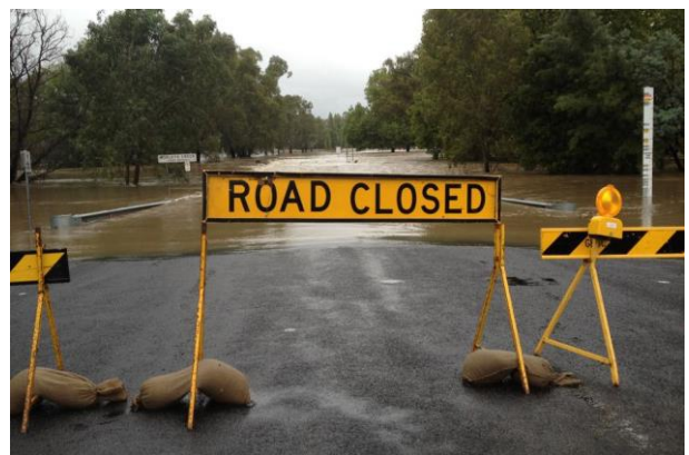
Photo 8 Yarri Bridge (4 March 2012)
